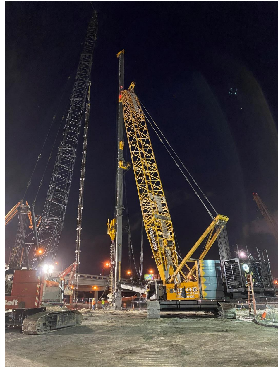
Crane with fixed lead system
